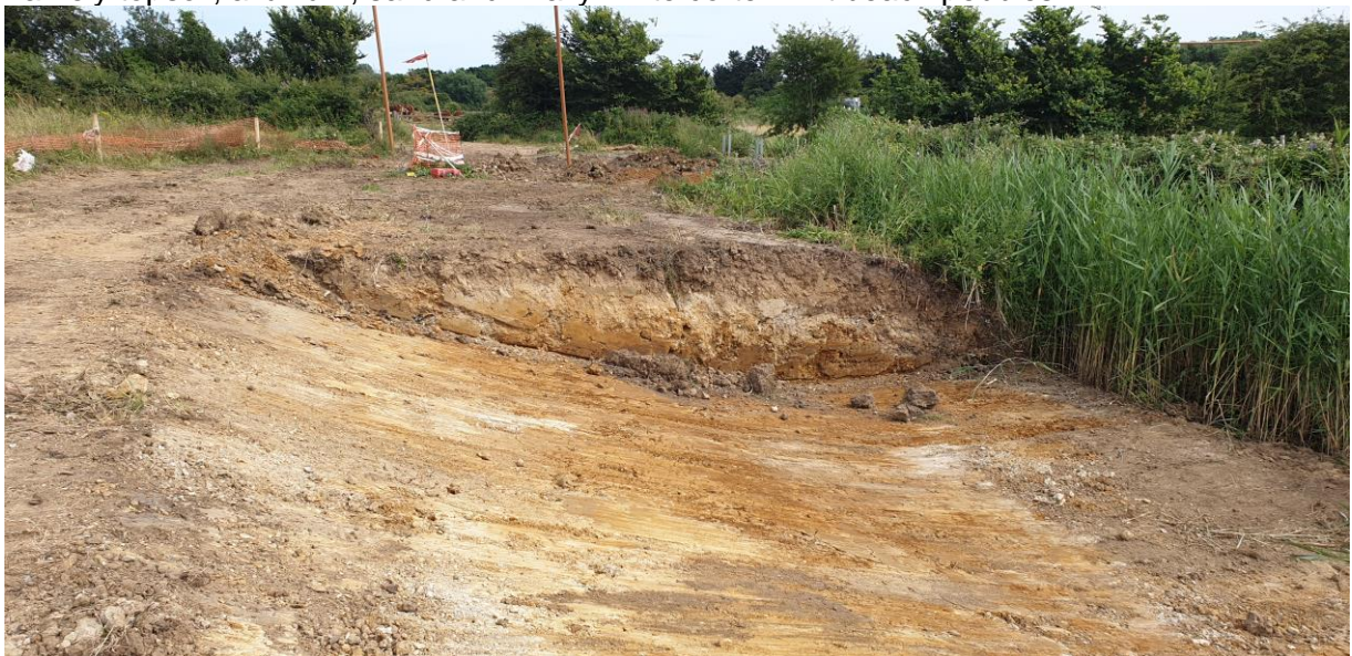
Figure 3 - Cutting the new river channel – view where the new and old channels will merge
