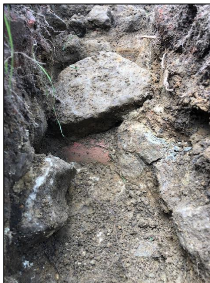
Figure 9: Image showing buried drain edge (Author)
