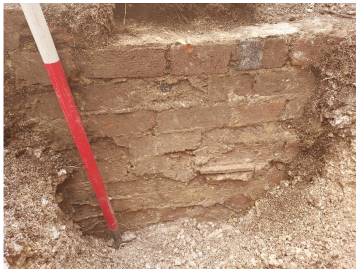
Figure 2 - Wall foundation with arch appearing bottom right
