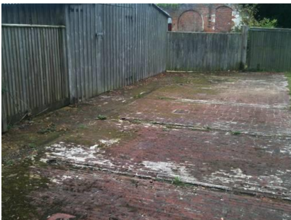
Fig.6 : Brick forecourt, old North Wing, showing stable floors and drains
