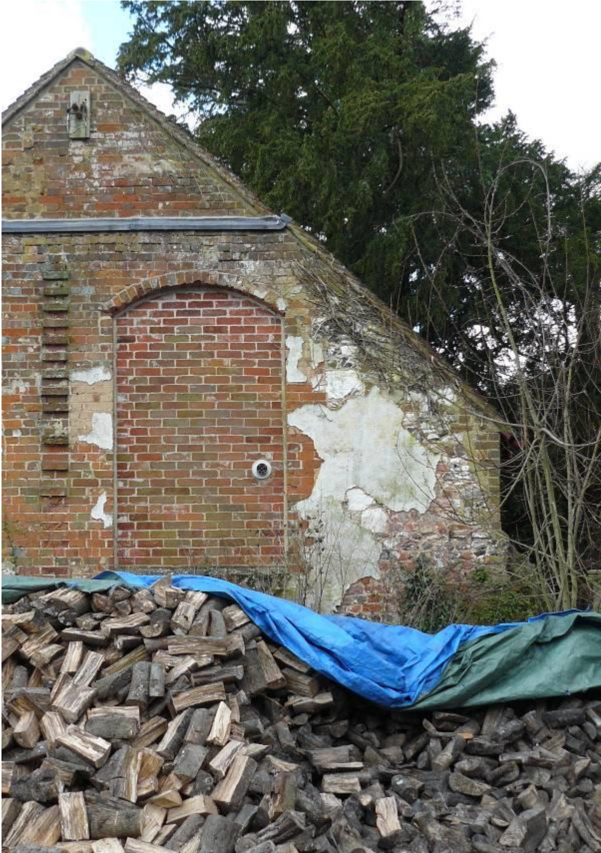
Fig.12 : Irregular build of NW corner at end of arcade
