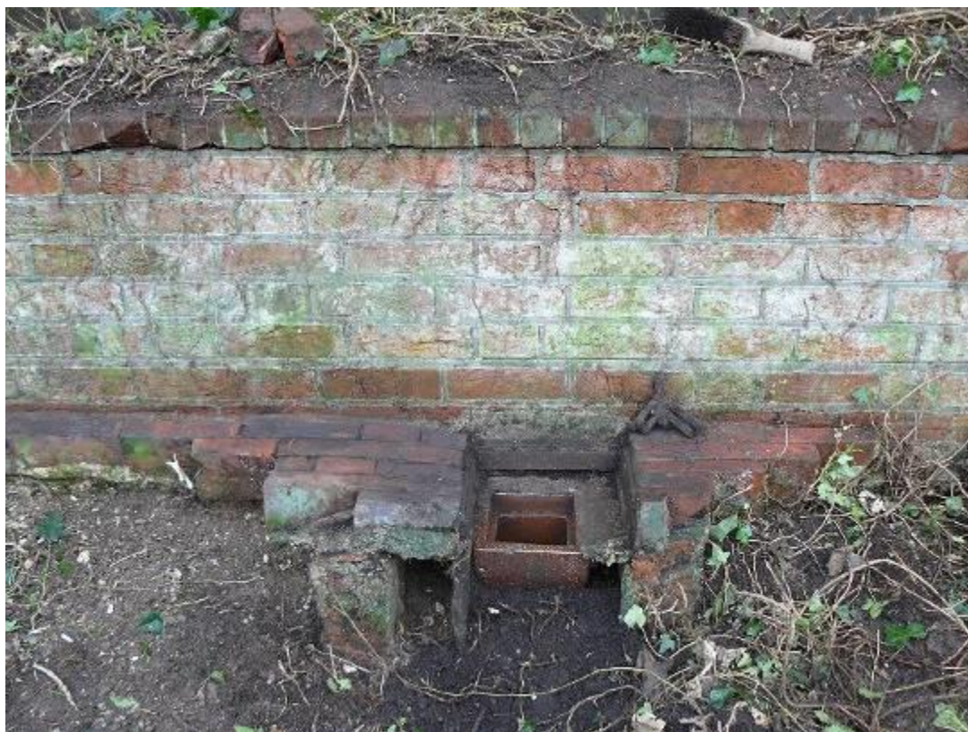
Fig.14 : Retaining wall, brick channel and gully on east boundary of site
