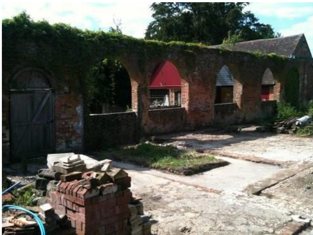
Fig.10 : The brick arches of the west wall showing concrete floors and partition walls
