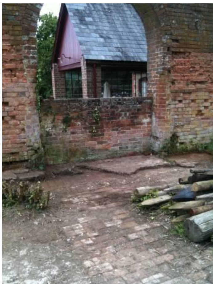
Fig.11 : Paved driveway from blocked up central arch, showing chamfered piers, concrete overlay and the trench carrying modern services
