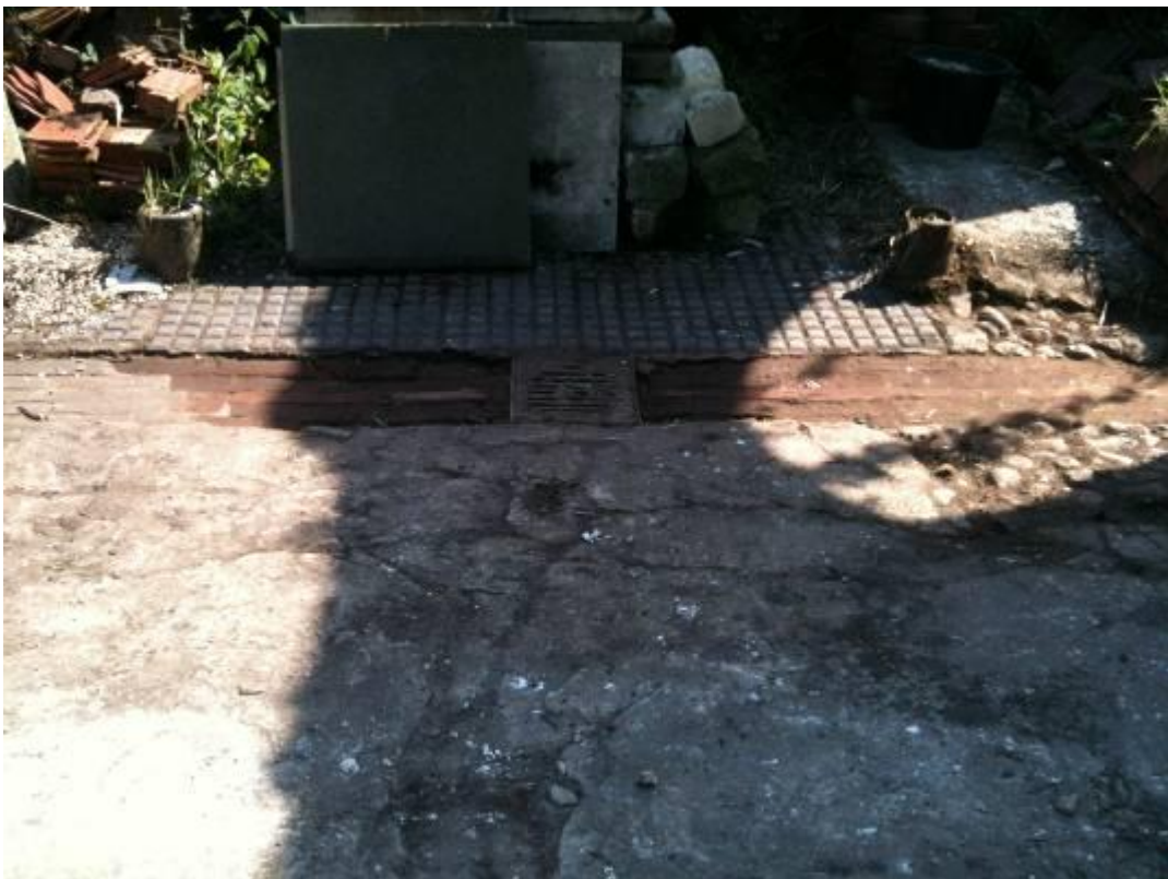
Fig.9 : South west corner showing chocolate block pavers, cobbles and stanchions
